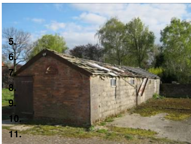
Foto 4: Te slopen stal
