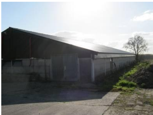
Foto 1: Te slopen stal
